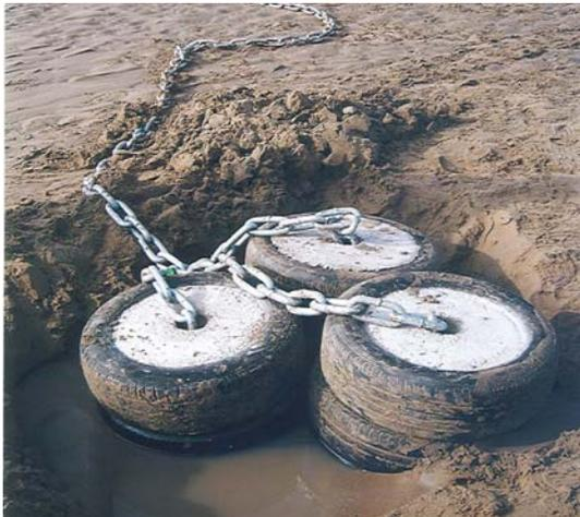
It was then simply a case of creating a sinker mass in excess of 500 kg by forming the sinkers into three towers of two and linking them with chain.
